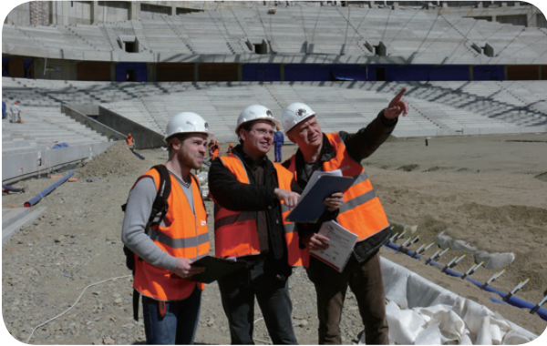
Huawei delivered its Indoor Connected Solution (ICS) to a football stadium in Russia.
