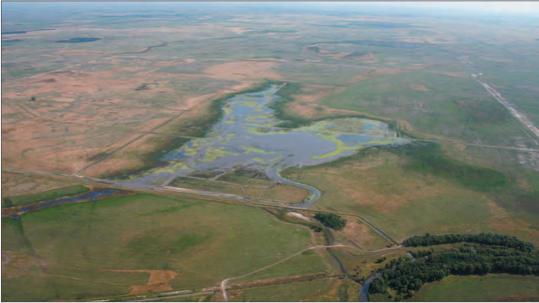
Plate 7.18 The flooded marsh after the completed works.
