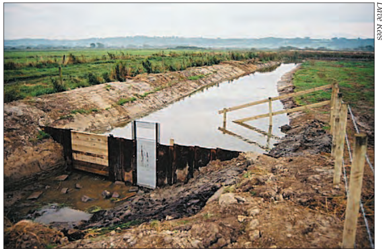
Plate 7.7 Completed trench sheet sluice.
