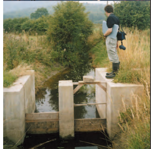
Plates 5.12–5.13 Pipe sluice (top) Dropboard sluice (bottom)
